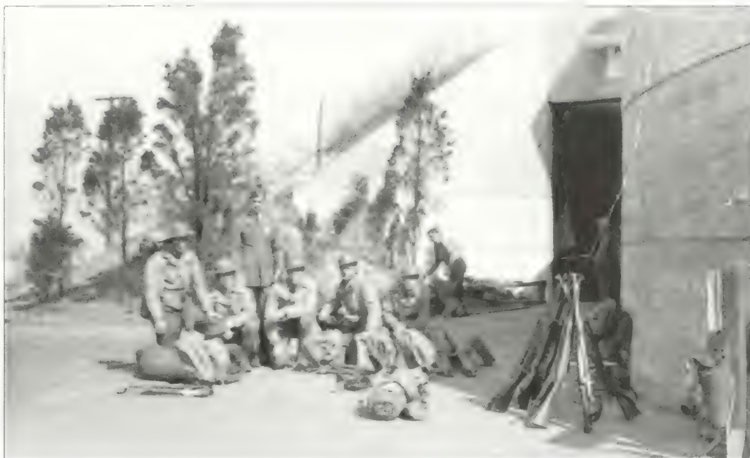
Figure 2.41. View looking northeast at entrance to covered passageway, Battery Kingman, circa 1940. A covered passageway featured standard-gauge railroad tracks embedded into concrete paving to accommodate rail deliveries of shells and gunpowder to the battery (GATE 8092).
